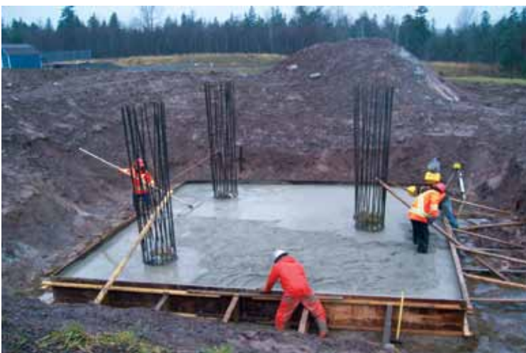
Town of New Glasgow, wind turbine foundation
