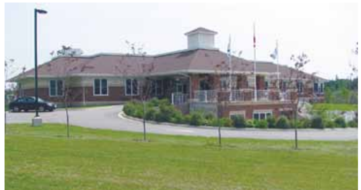
Yarmouth District Administration Building
